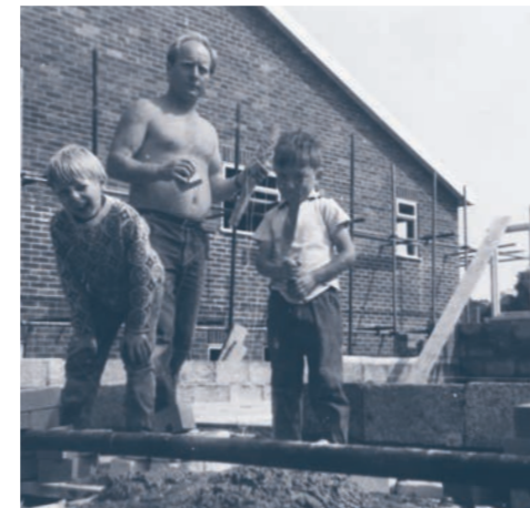
Pat & George Truelove, founding members of Truelove Property & Construction LTD on one of their first builds
